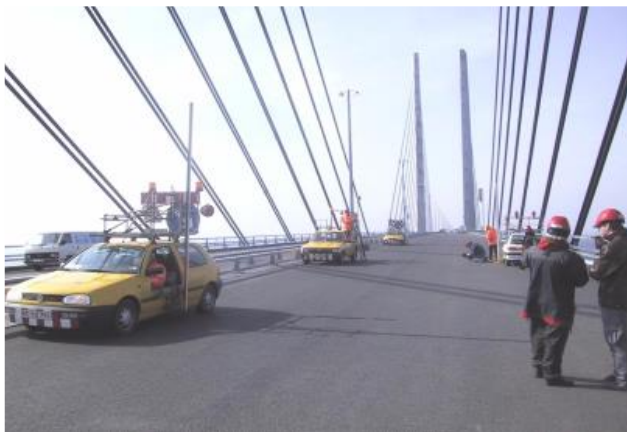
Fig. 3 Performing measurements by motorized levelling with three cars (Oresund Bridge, 2000)
